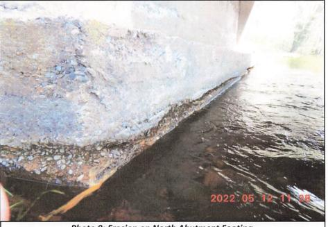
Photo 9: Erosion on North Abutment Footing
