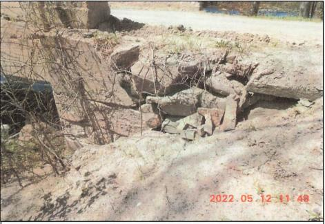
Photo 7: Seperatory Cracking, Scaling, and Tilting on Northeast Wingwall and Failed Retaining Wall
