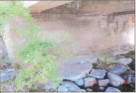
Photo 3: Scaling and Cracking with Efflorescence on North Abutment Wall
